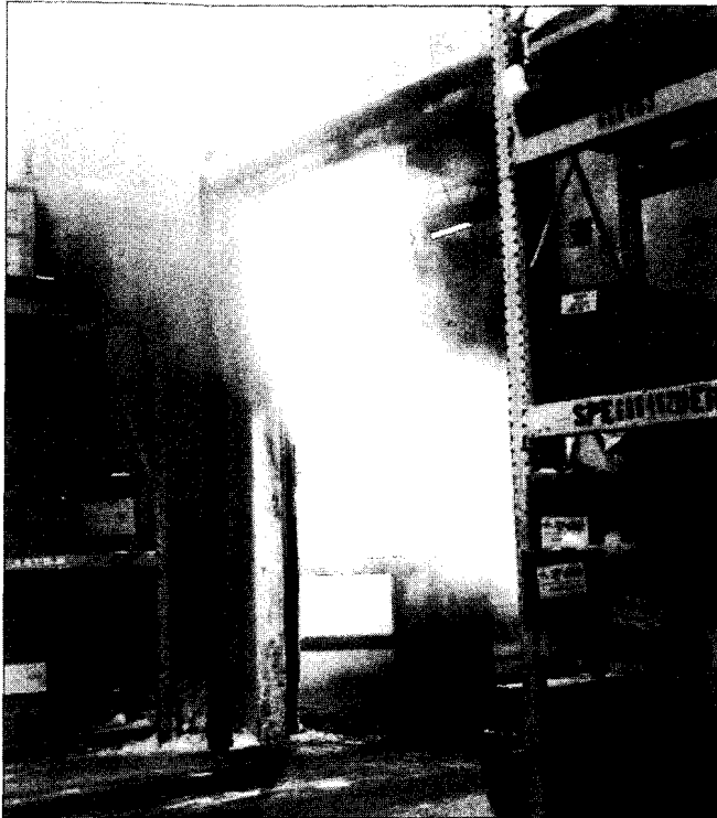
Figure 1 Gravitational and psychrometric effects. Airborne ice-crystal infiltration as seen in the field can be seen beforehand in the office on a psychrometric chart.
